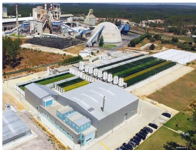
Figure 1 - Allmicroalgae S.A. facilities, Pataias 2
